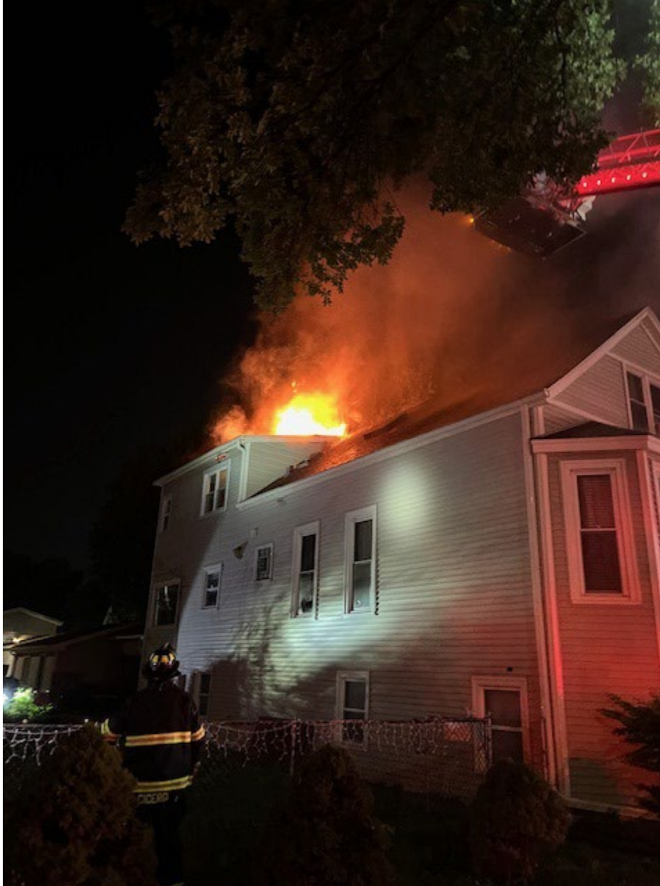
Smoke and fire showing on arrival of FPDF
