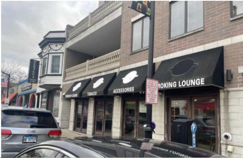
Photograph 3 View: Alternate Exterior Photo Taken: 11/12/24
