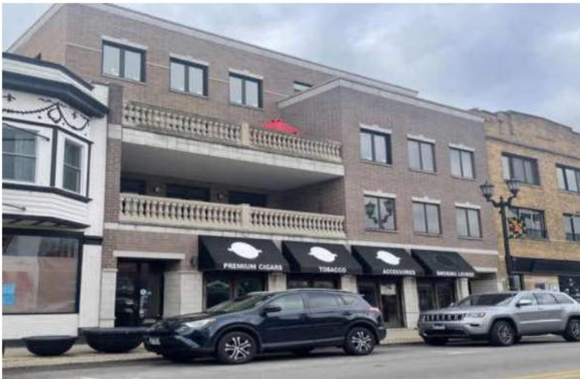
Photograph 1 View: Exterior Project (subject is ground retail unit) Photo Taken: 11/12/24
